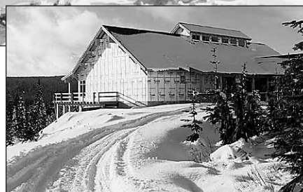
The west side's new lodge, currently at the lock-up stage, is scheduled for completion next summer.
