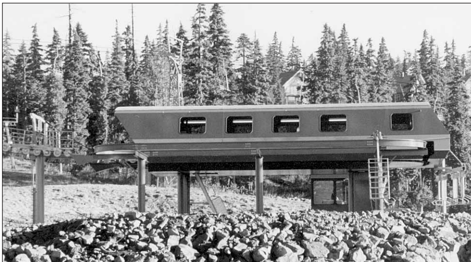
The Hawk High Speed Six Pack is ready to whisk 2400 skiers and boarders per hour to the lower West Basin, increasing intermediate terrain dramatically.
