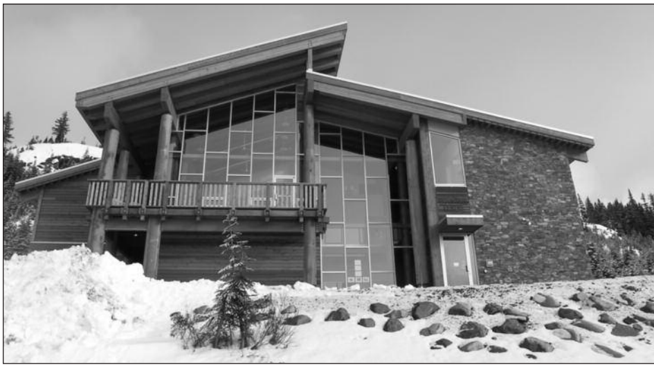
Mountain Centre accommodation facilities include a series of dorm rooms that can sleep 40, washrooms with fully accessible showers, a dual kitchen and meeting spaces. Photo by Neil Havers
